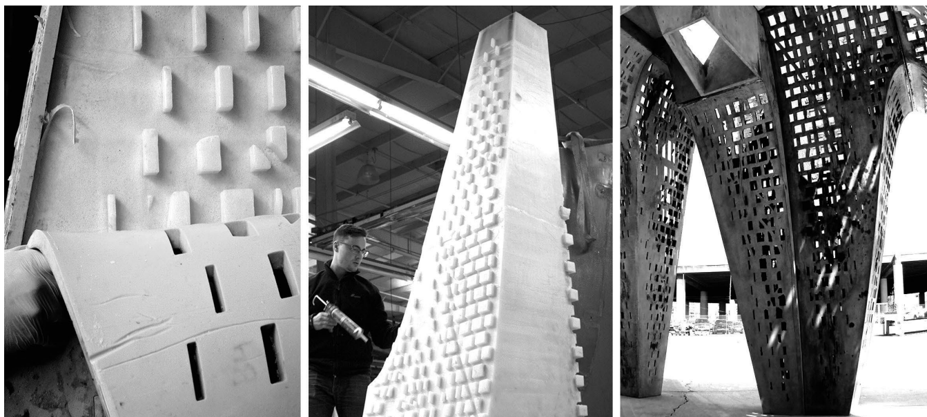
Final casting process of 'wax on / wax off' method with, a. peeling away silicon inlay once wax is cast, b. final wax formwork prior to casting the concrete, c. final columns with pattern as void (Photographs by author).
